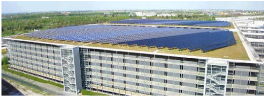
Figure 1: Roof top PV system - Car park at the Munich fair center in Munich-Riem, Germany. Source WIP-Renewable Energies [1]
